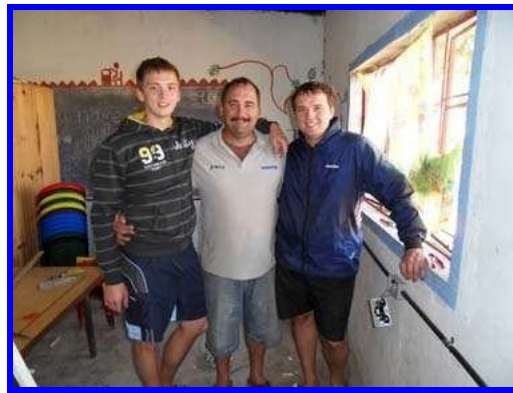
Gert and sons installing electrics
