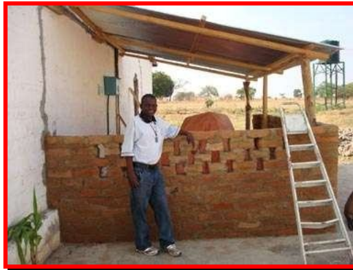
Building work continues on site
