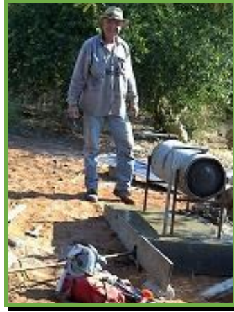
Lourie busy installing the "donkey".
