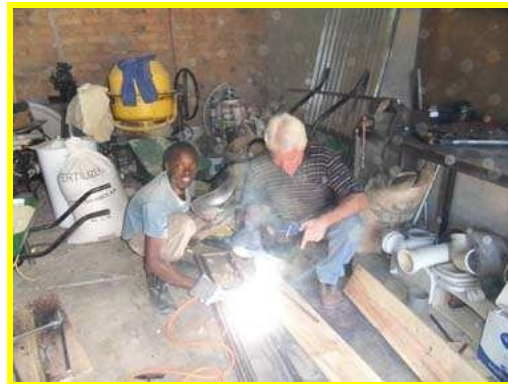
Welding of the benches
