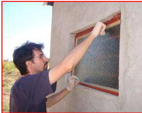
Nico – sit die badkamervensters in / fitting the bathroom windows
