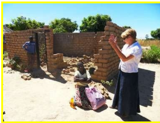
Burnt down house of a widow
